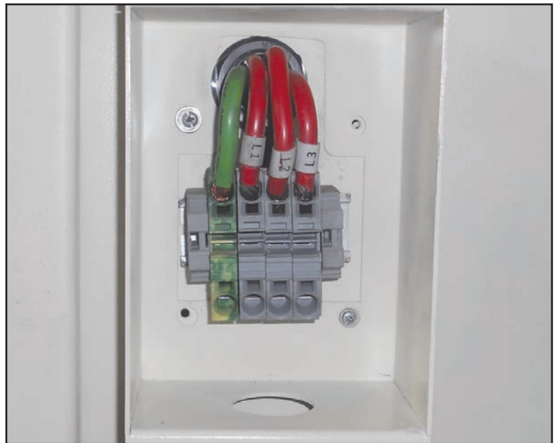
Figure 67. W1773 power junction box.
