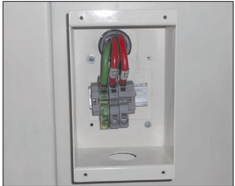
Figure 66. W1772 power junction box.
